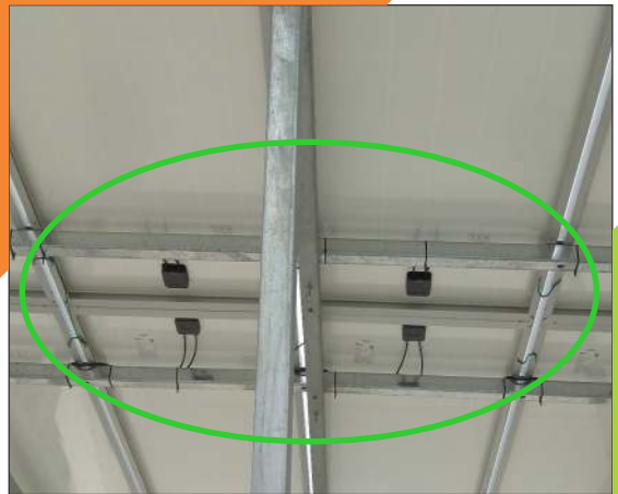
Use of UV resistant cable tie which is more durable than normal cable tie.
